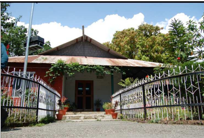
Front View of Principal's Office and Administrative Block
