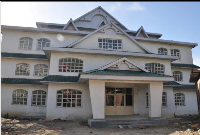
College Auditorium, under construction
