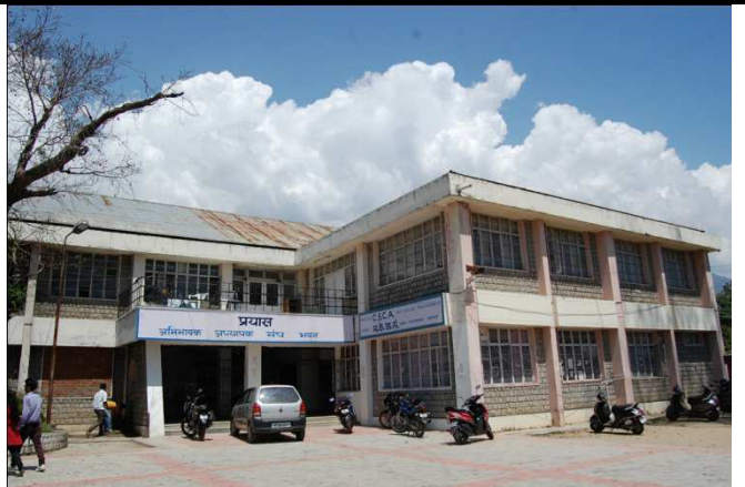
Front View of Multi-Purpose Hall
